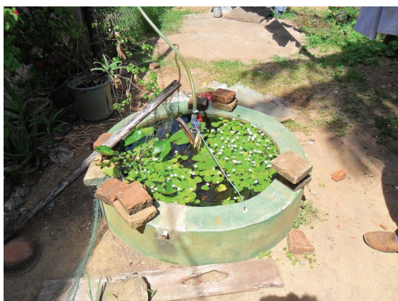
This biogas digester supplies gas for cooking to two homes in Sri Lanka from kitchen scraps. The water over the dome helps to prevent cracks in the surface. Photo courtesy of HELP-O.
