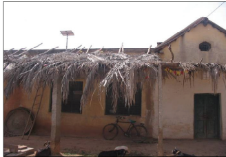
Solar panels atop the cocoon rearing centre.
